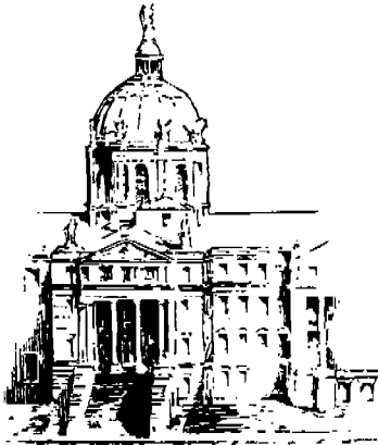
McLennan County Courthouse
